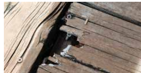
Shown Above: Ipe (Brazilian Walnut) Hardwood decking installed with face driven screws.
