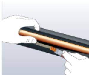
3. Place the slit tube onto the clean pipe; apply a thin, even film of Armacell 520 adhesive to the two cut edges using a short bristle brush. Apply the adhesive along the tube length. Alternate 6-8" on both sides to maintain even tackiness.
