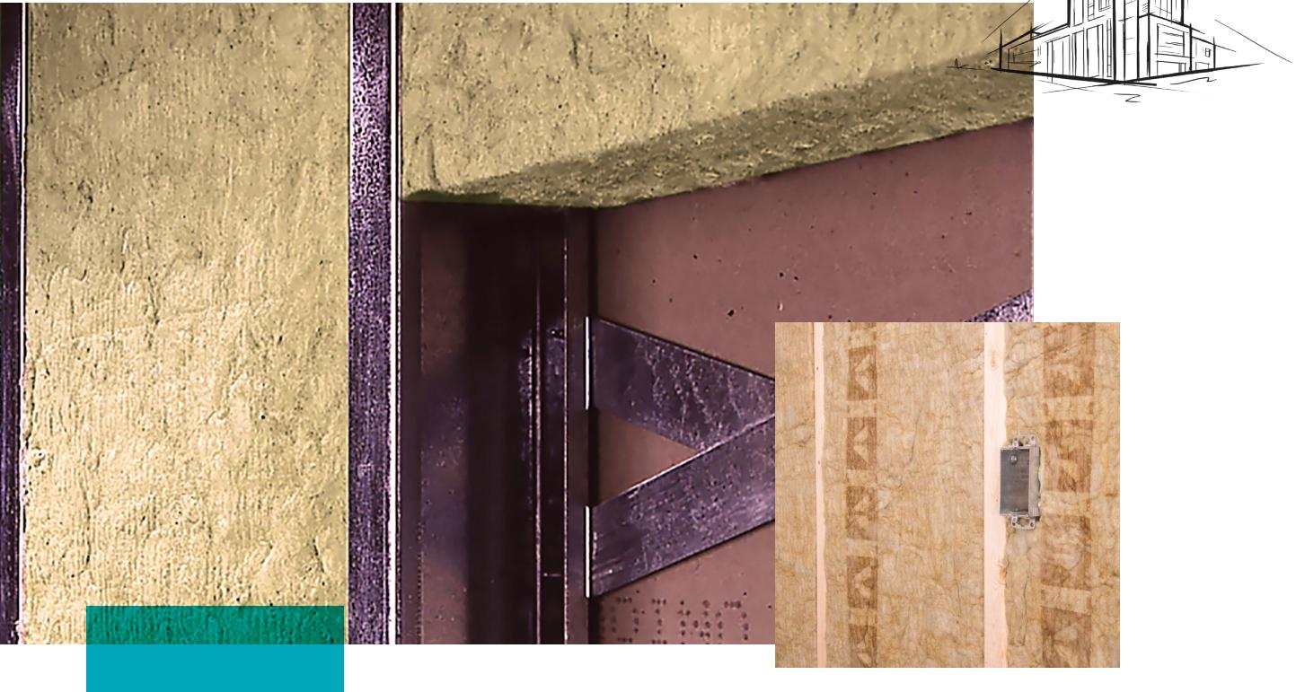
ROCKWOOL AFB® is a lightweight, acoustical fire batt stone wool insulation specifically designed for steel stud and wood stud interior wall and floor applications. Its superior sound absorbtion and fire protection contribute to the overall comfort and safety of occupants.
