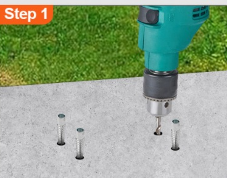
Determine the installation holes and drill.
