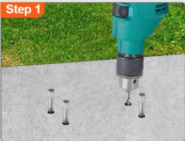
Determine the installation holes and drill.
