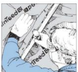
Fit the end of the insulation snugly against the top plate at the beginning of the cathedral ceiling framing. Work upward until the cavity is filled.
